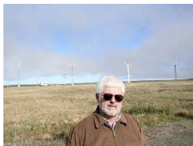
The Kotzebue Electric Association operates 17 wind turbines, which last year generated 7 percent of Kotzebue's electricity. Photo/Amy Schenck/For the Journal
